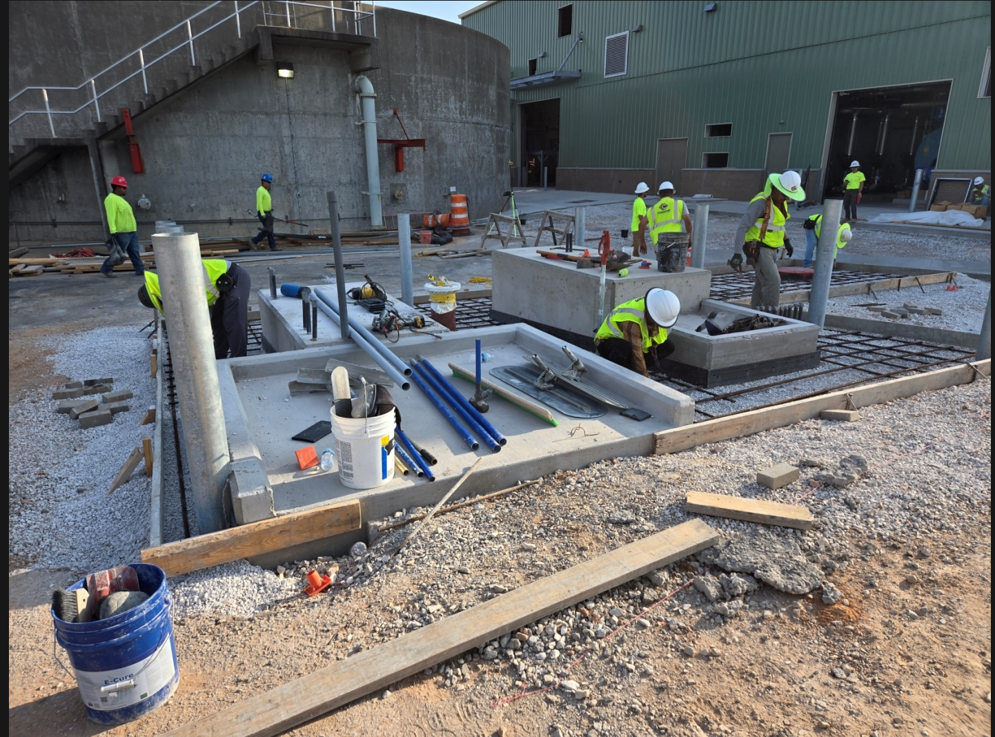
Preparing formwork and rebar for slab pour at septic receiving station
