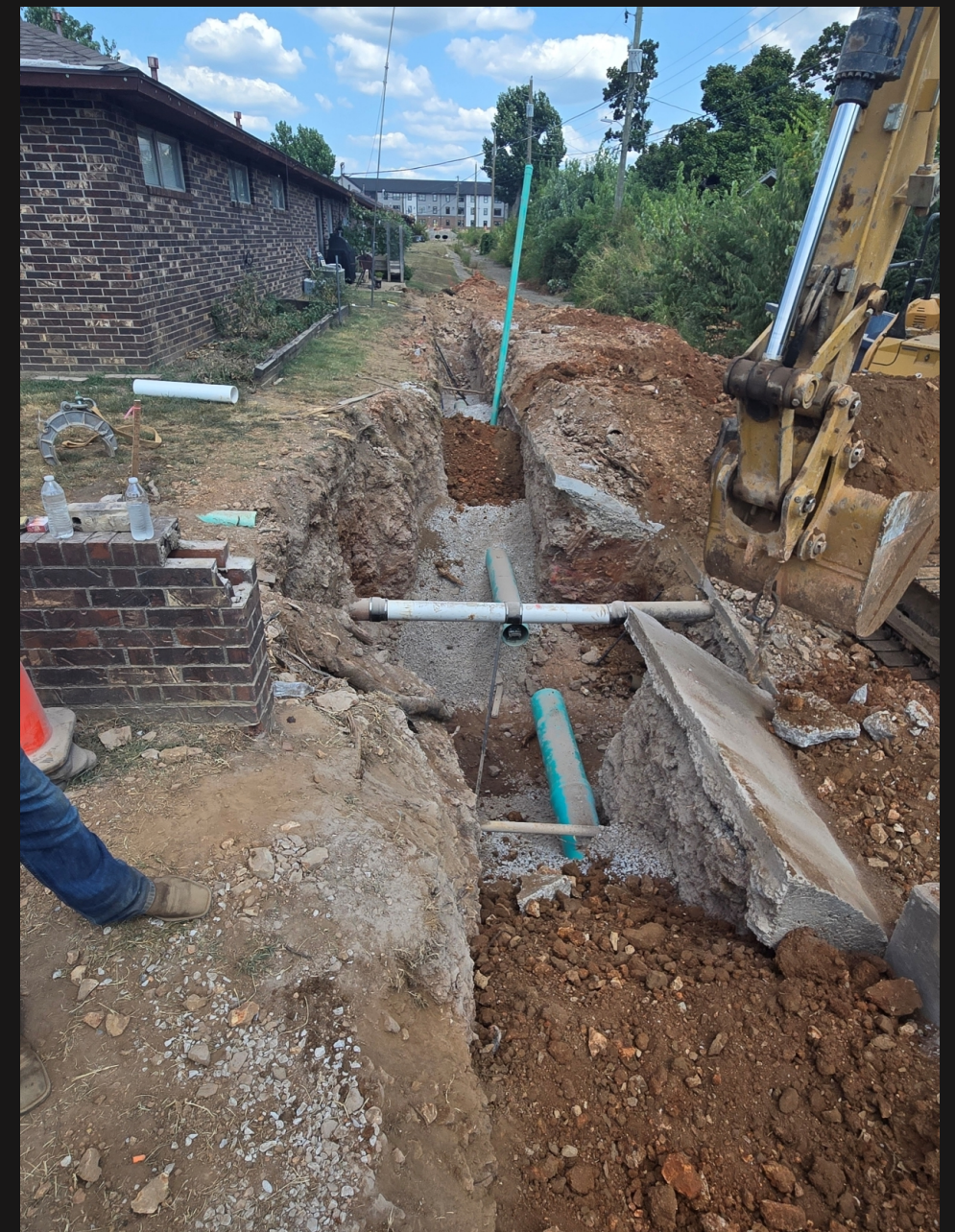
Looking east along the sewer alignment from Rife Dr., just south of Walnut St.
