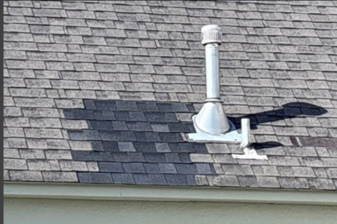
Proposed shingle next to old shingle
