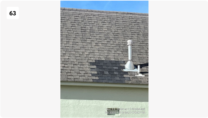
Project: Sasha/Bruce Thompson B22 Date: Dec 11, 2025, 11:30 AM Creator: Josh Miller
