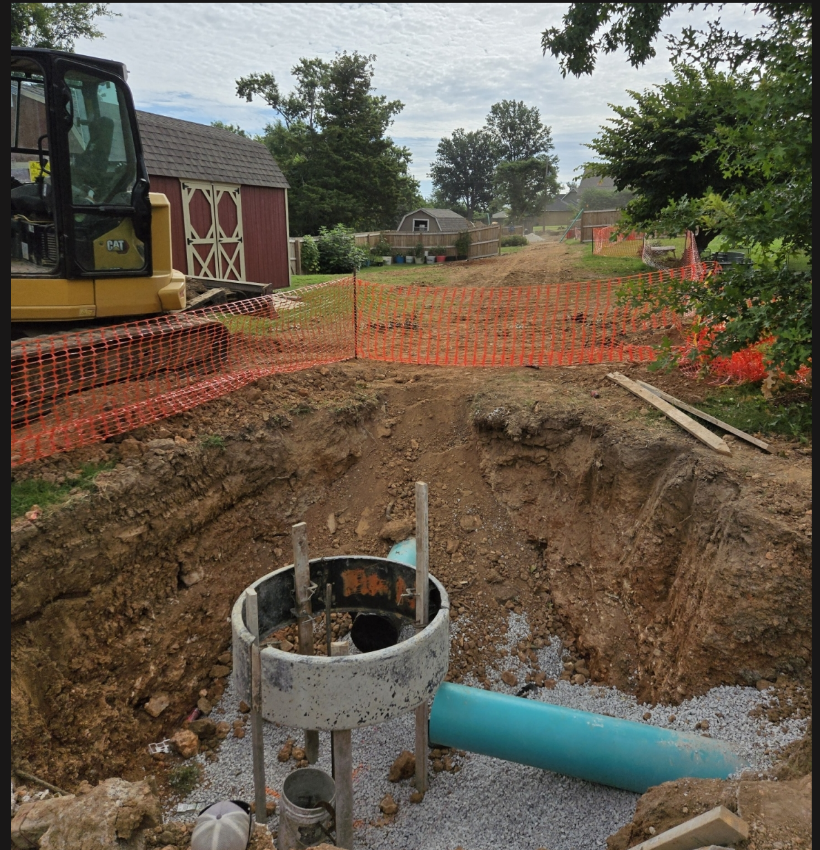
Looking east along the sewer alignment through backyards along Chateau Dr.
