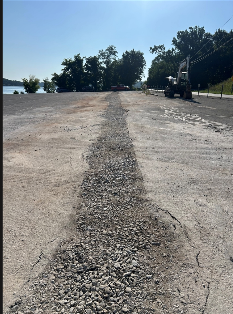
Completed section of water main installed at the boat ramp parking lot just west of Hwy 12 bridge.
