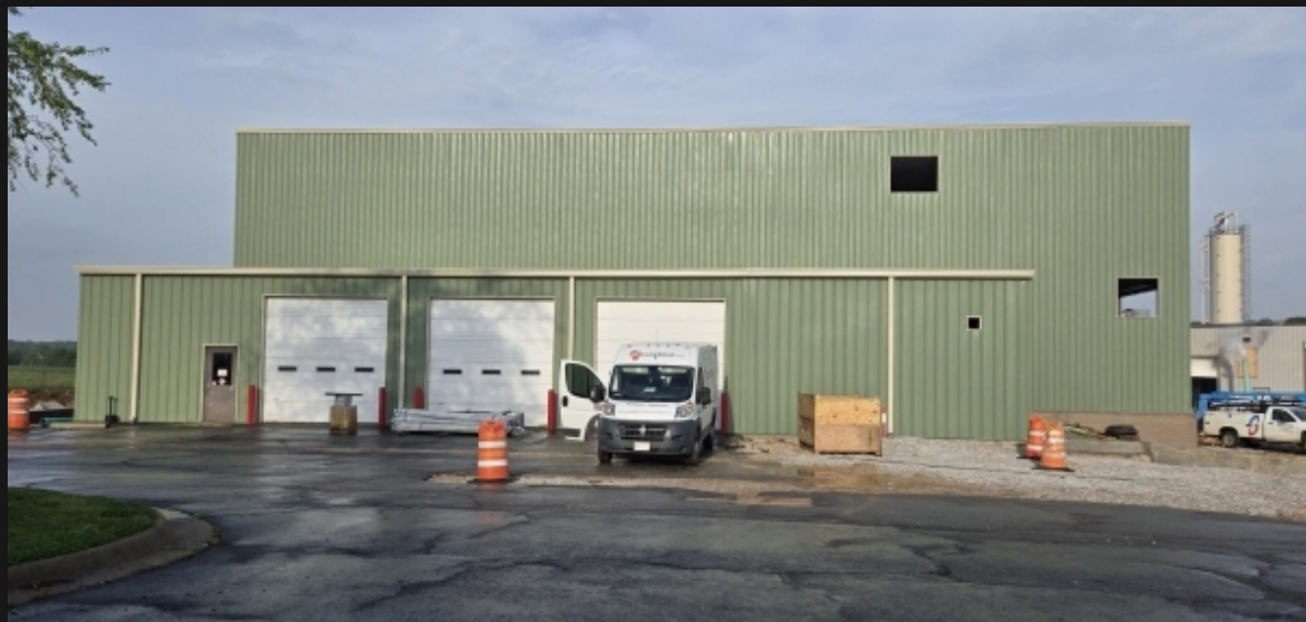
West Face of Existing Building
