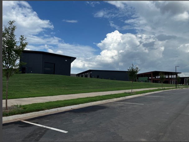
View from S 31 st Street
