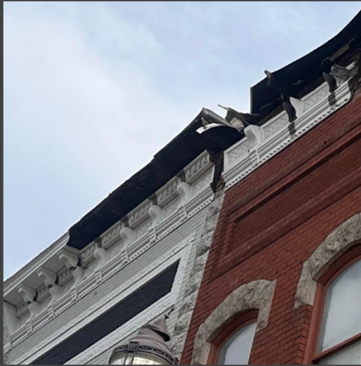
Close up of Cornice
