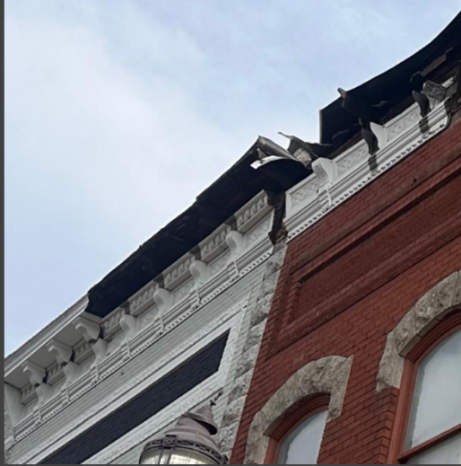
Close up of Cornice
