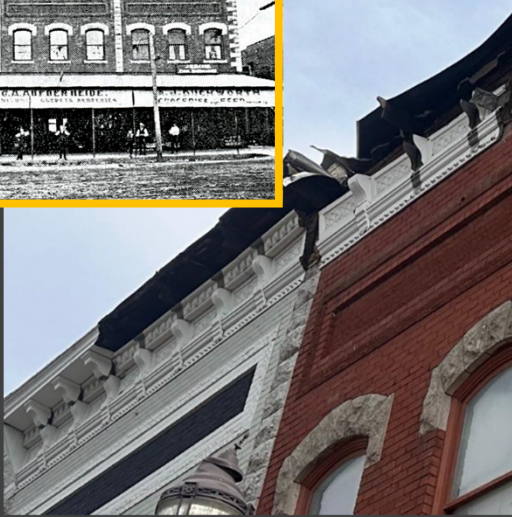
Close up of Cornice
