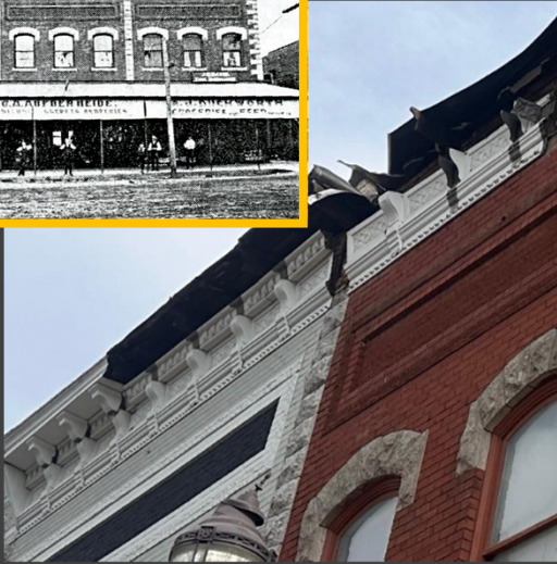
Close up of Cornice
