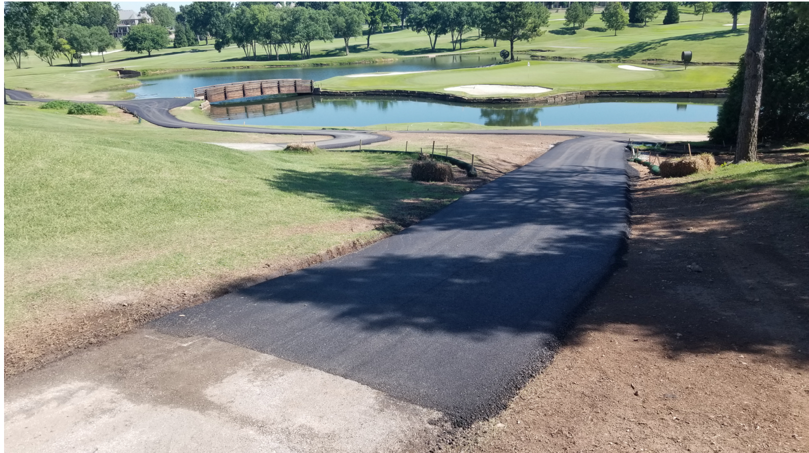
Photo: Asphalt cart path repairs near the clubhouse on 6/12/24.
