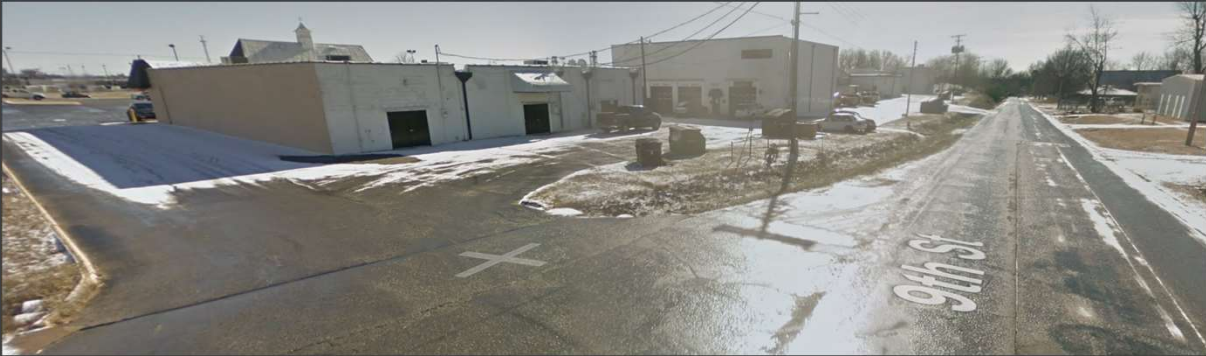
Looking South – 9 th Street
