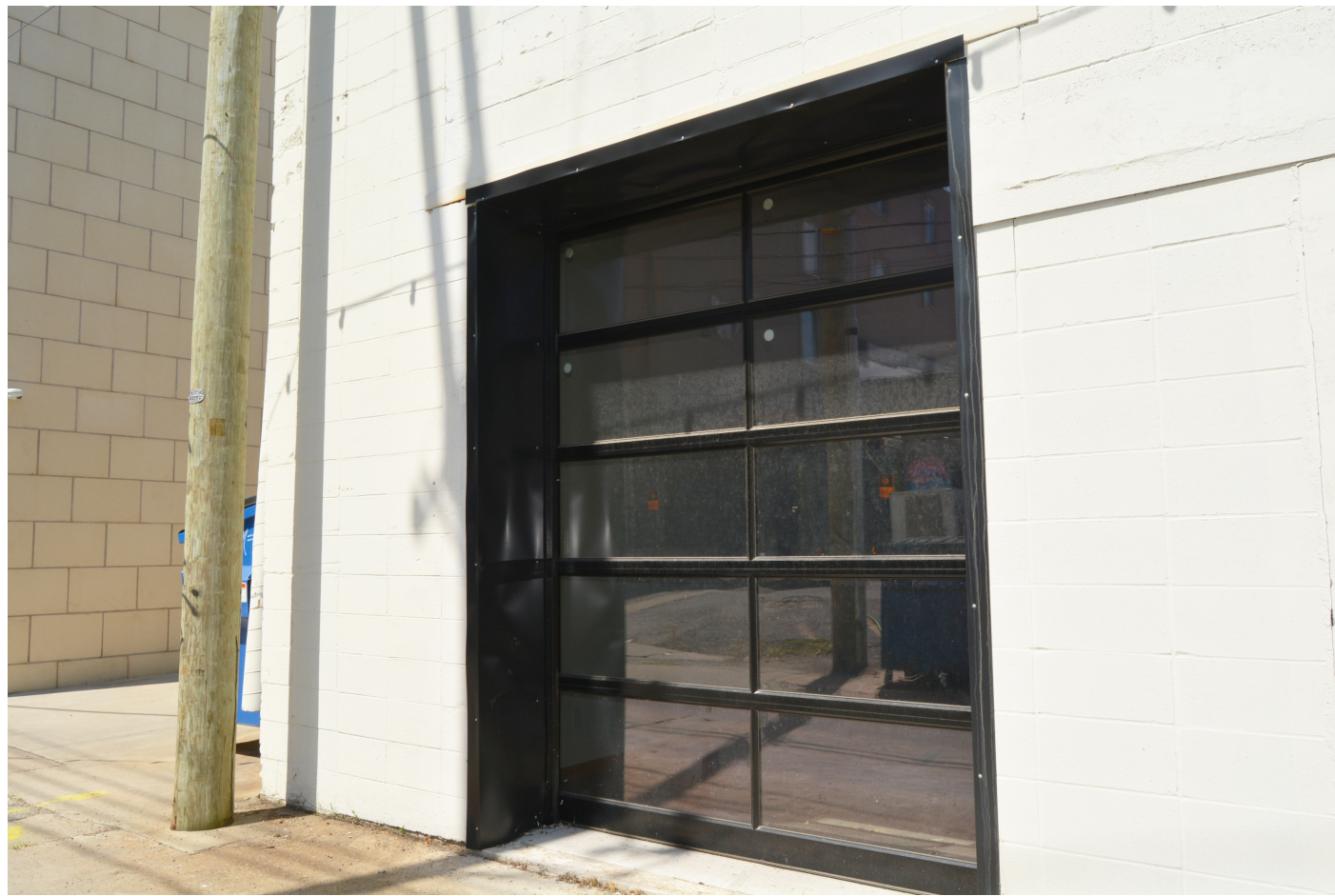
7 EXISTING PHOTO - OVERHEAD DOOR NOT TO SCALE
