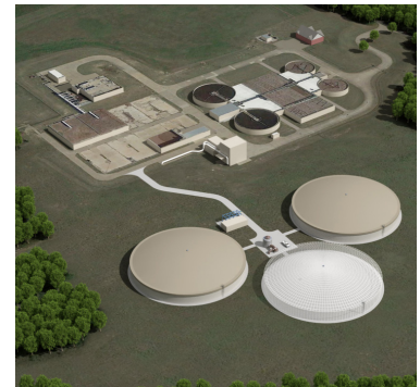
21-MG covered storage concept for TRA ROCRWS (in construction now)
