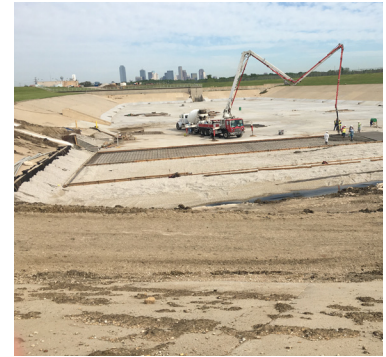
180-MG DWU peak flow storage renovation
