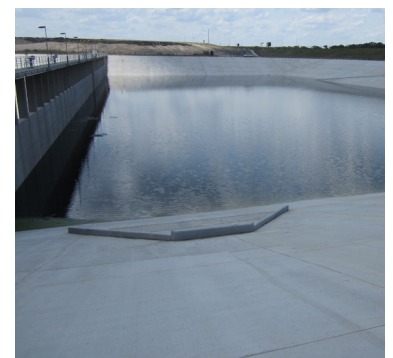
160-MG peak flow storage at TRA CRWS
