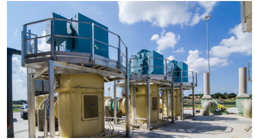
450-MGD DWU Raw Wastewater Lift Station
